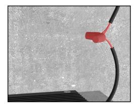
5. Feed low voltage wiring to the bracket and lift the fixture board assembly to the low voltage electrical connection and make the connection.
