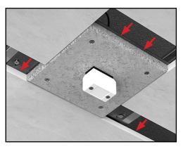
9. Cut and install the drywall around the fixture, ensuring that the fixture board assembly is flush with the surrounding drywall. This will allow a finish of one eight inch of plaster around the finishing guard.
