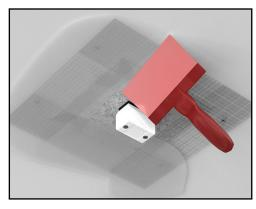
14. Allow for the tape to dry and apply your first coat of plaster to the tape seam, lightly skim coating the surface of the fixture board assembly.
